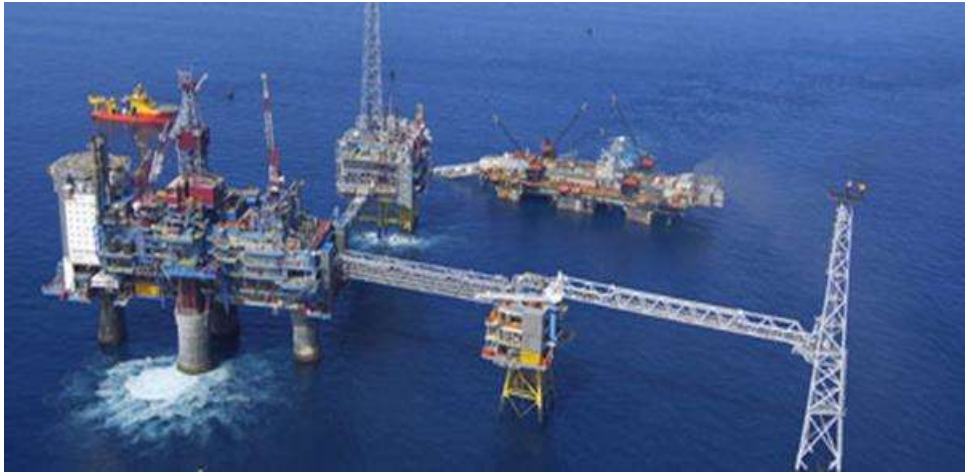
Fig 2.8.1 Aerial view of the Sleipner platform
